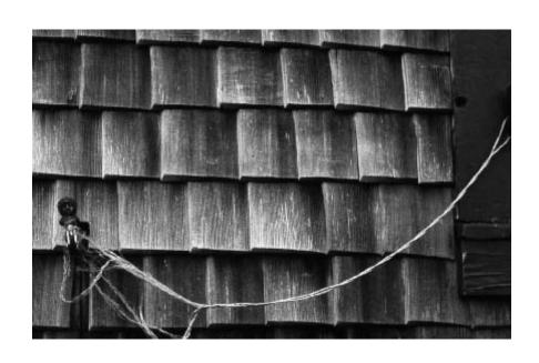
17. Externally, walls are clad with timber shingles in equal courses, lapped in two directions.
