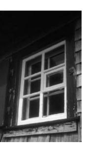
36. The hut's windows have two layers of glazing, both of which open for variable degrees of ventilation. Some windows—like this one to the dining area—also have an additional small opening light in the outer leaf.
